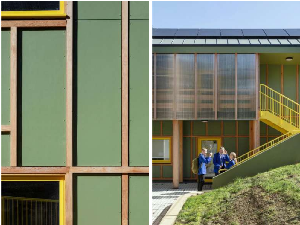
Detail of the timber battens on the facade and pupils relaxing during breaktime. Photos by Rachel Ferriman.
